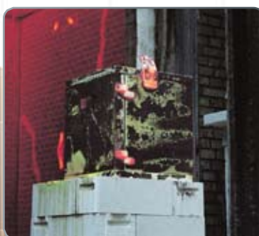
Removal of cabinet from oven
